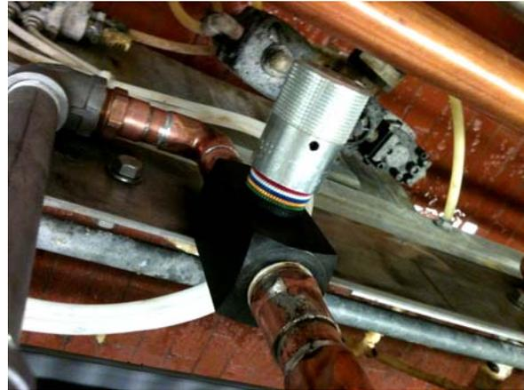
Figure (6) Flow regulators installed at each dispense head to change the flow of water in each sheet-pan.
