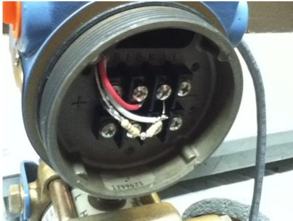
Figure 6: Resistor in line with 4-20ma output to get a voltage signal
