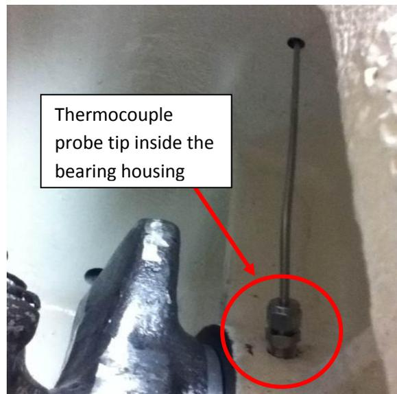
Figure 3: Installed crankshaft bearing thermocouple probe
