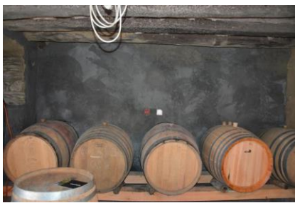
Biochar clay plaster in wine cellar helps control humidity.
