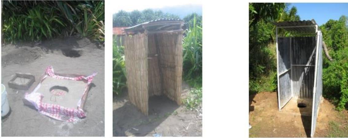
**Figure 2: Conventional arborloo concrete base (left), low cost conventional shelter (middle), and improved shelter (but too expensive) (right).**
