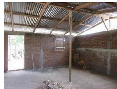
Current roof design with the exception that 4 Walls has since switched to metal C channel trusses instead of wood beams (which are welded together on-site).
